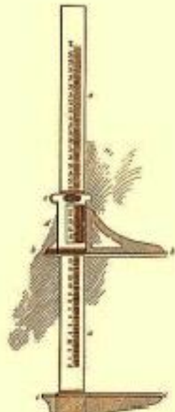
FIGURE 2. SLIDING COMPASSES.
