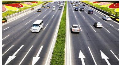
Figure: Traffic control
